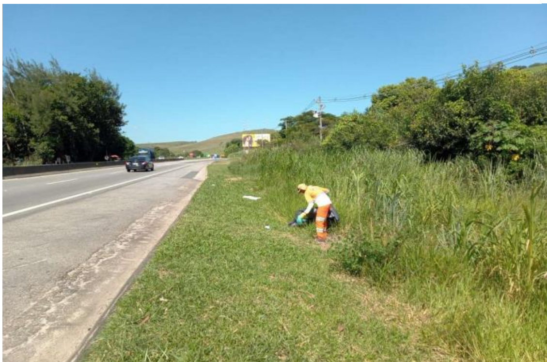
Figura 6.10 Via Lagos – Cata Cata– Km 14+000 Norte
